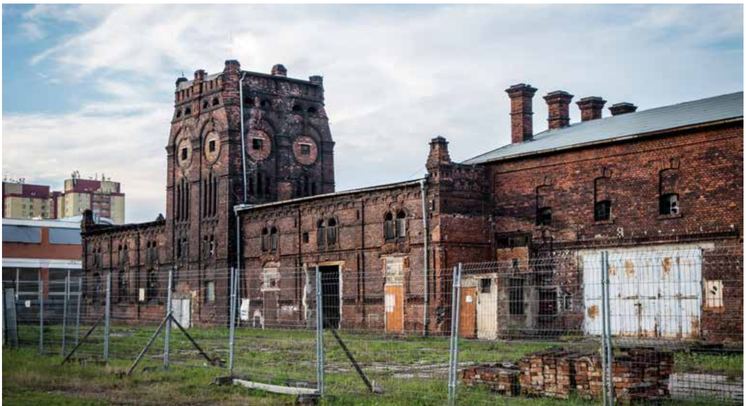
Neutěšený stav budov. The buildings have become derelict.
